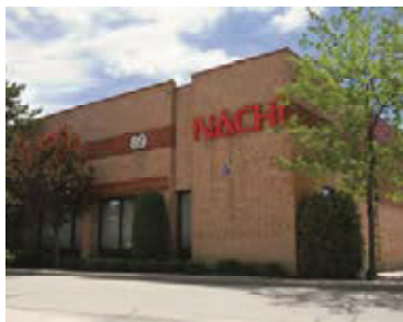
Sales Office & Warehouse, Concord, Ontario, Canada
