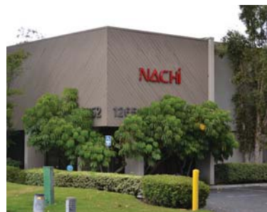
Sales Office & Warehouse, Cerritos, California
